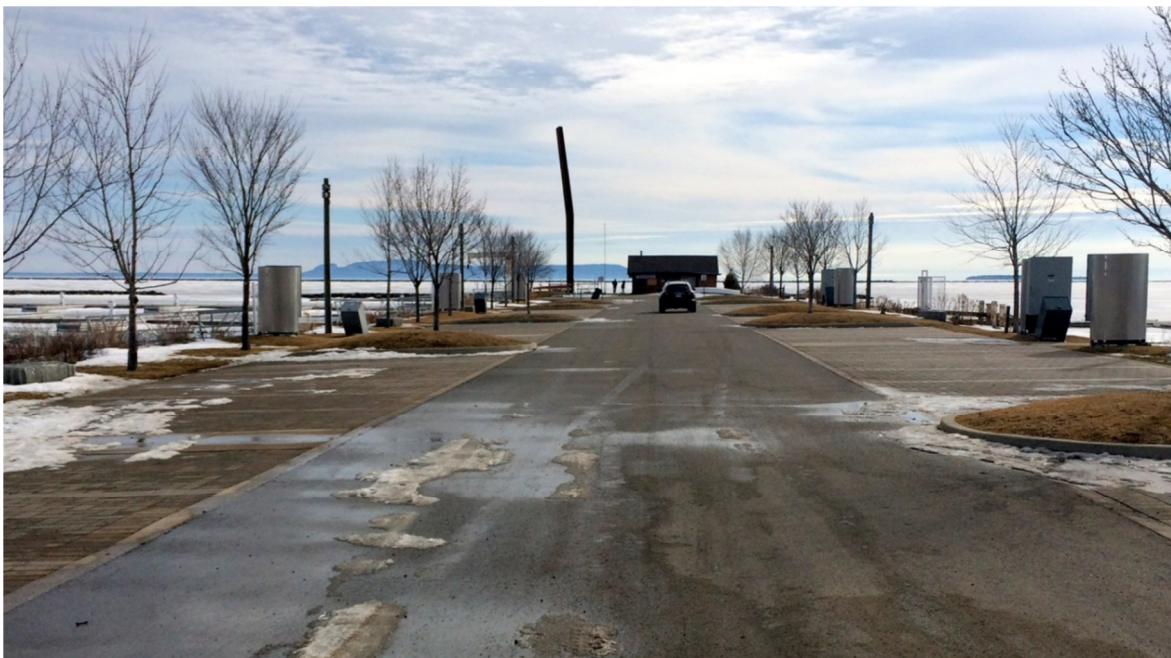
Above, view of Pier 1 parking facilities with 11 “bump-outs” jutting into the lot.
