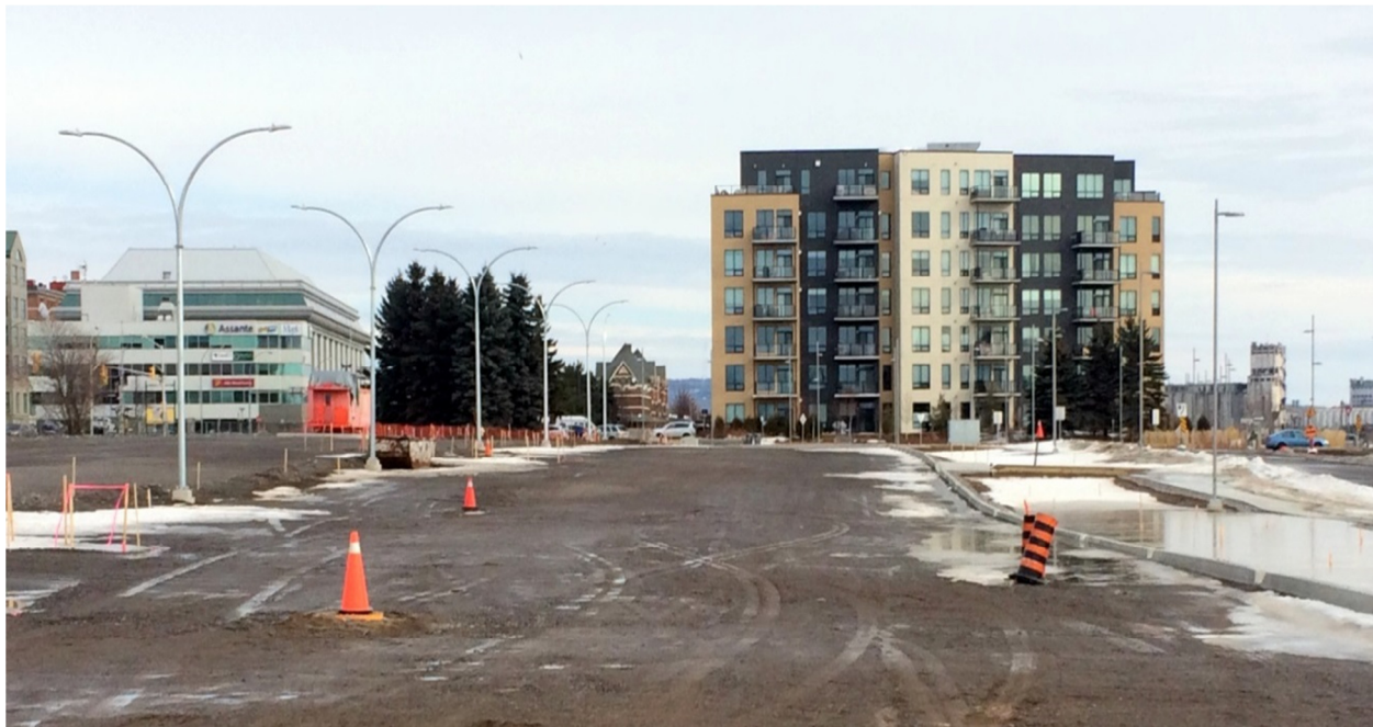
Above, new parking lots currently being developed in the area west of the Boater Service lot and north of the pumping station. Curbing is in place along the eastern perimeter of the lot.
