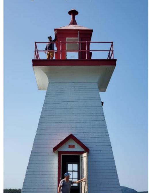
No 10 Lighthouse opened up for access work
